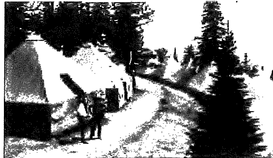
Completed camp segment, July 1934. Photo SP10-7.
